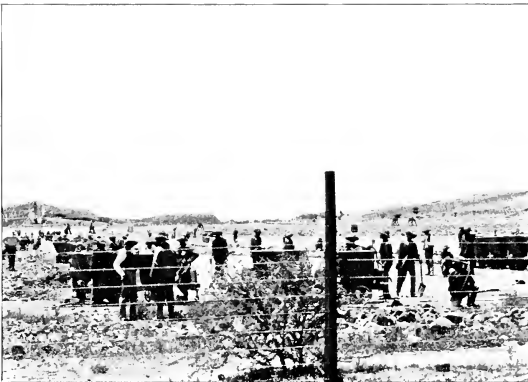
10.—The Depositing Floors.
